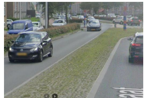
Figuur 2: Grasbetonstenen in middenberm.
